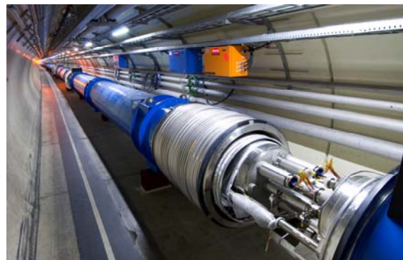
LHC Assembly in the tunnel
