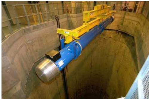
Lowering a Dipole into the tunnel
